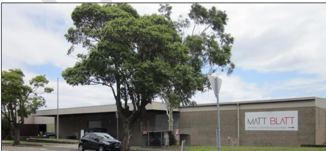
Figure 5: 141 Allen Street – Flood Street frontage looking northwest
